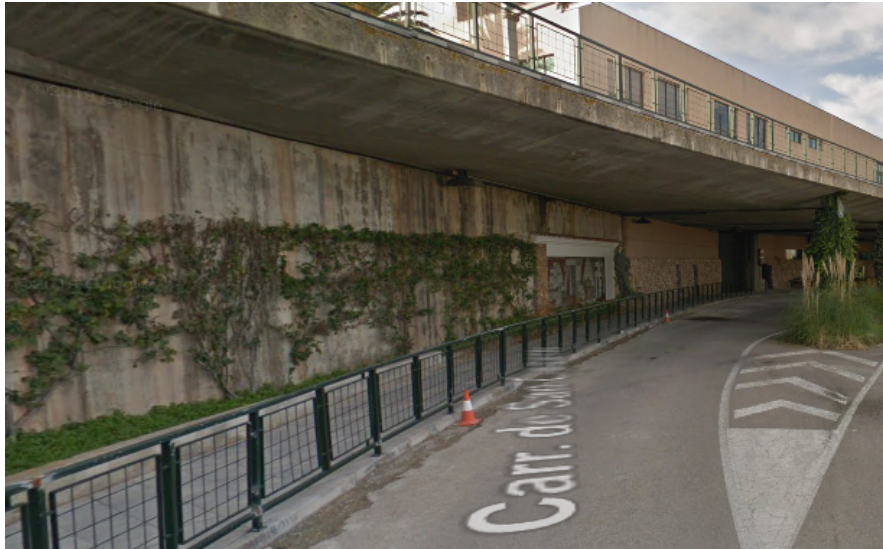
Figure 28: View of the span (section 3)
