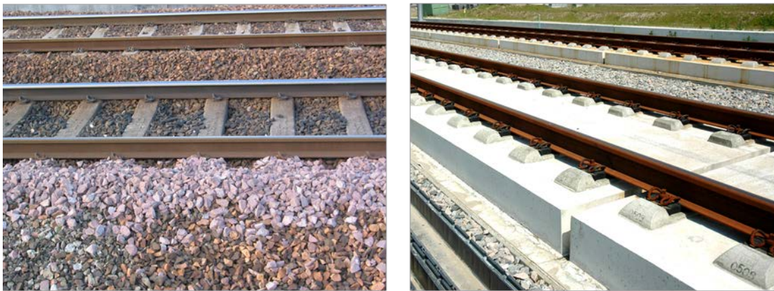
Figure 2. Ballast and concrete track beds. Sources: [28, 29].
