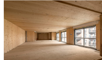
Imagen 4.11 Vista interior durante la construcción. - https://www.architectsjournal.co.uk/buildings/high-density-low-carbon-dalston-works-by-waugh-thistleton
