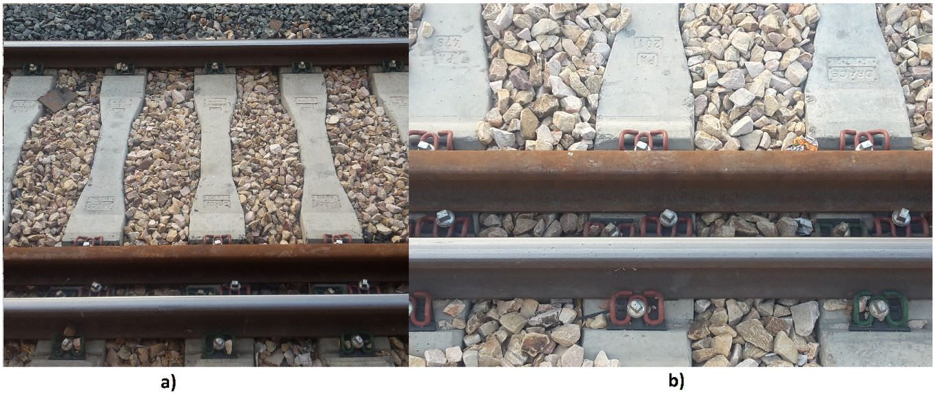
Fig. 3. View of dual gauge railway track (a) and detail of rail fasteners at the double rail side (b).
