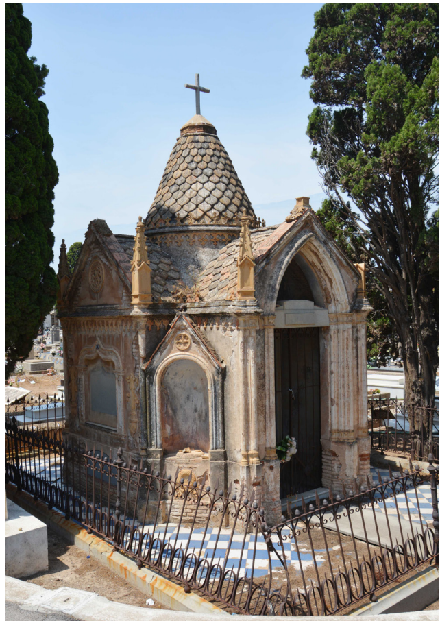
Fig. 40_ Exterior view of the chapel. Ph.: author
