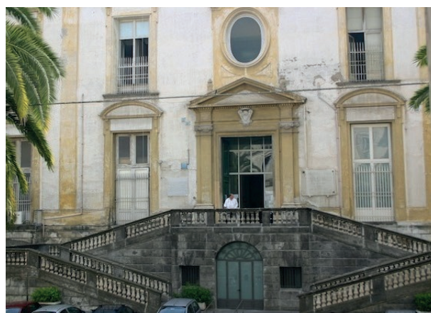
Figure 1 | The main facade of the Hospital of Incurables. Source: https://www.napoligrafia.it/monumenti/complessi/incurabili/incurabili01.htm
