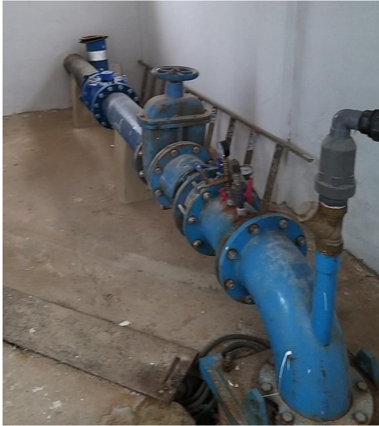
Figure 8: Extraction Pou del institut
