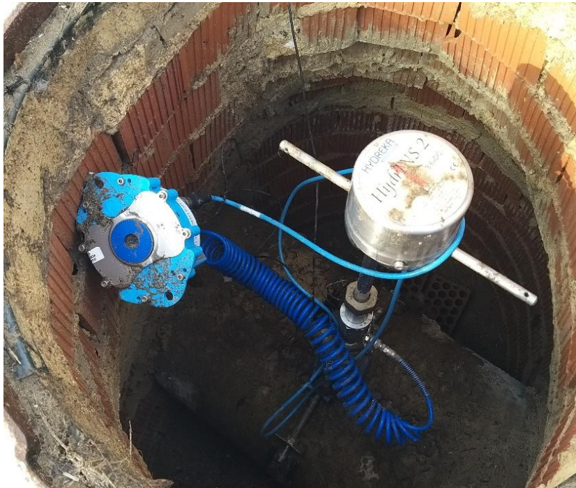
Figure 14: Insertion flow meter
