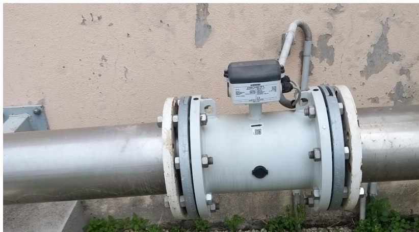
Figure 15: Electromagnetic flow meter
