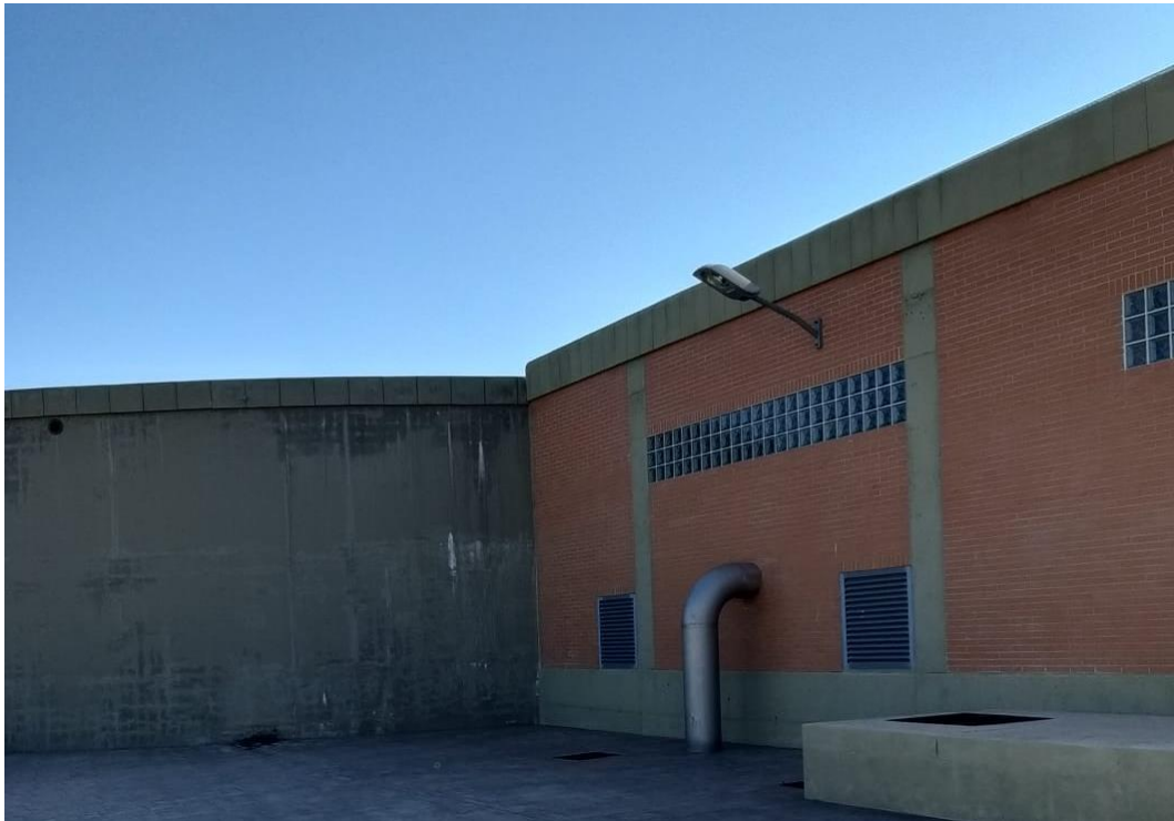
Figure 5: New reservoir in Mareny de Barraquetes
