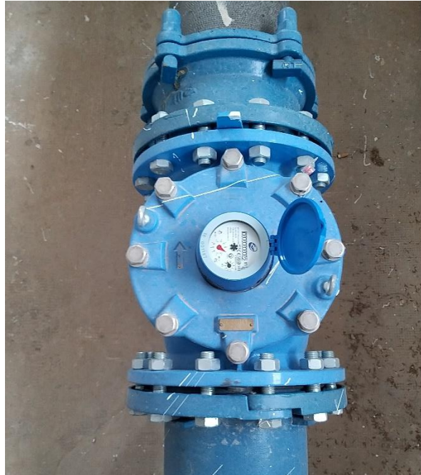
Figure 16: Mechanical flow meter
