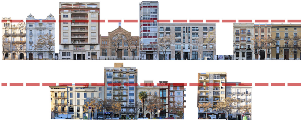
Fig. 2. Photograph of the facades in Blanquerías Street, with an indication of the required cornice height. The buildings that exceed this height must be replaced under the terms of the Special Protection Plan (PEP).
