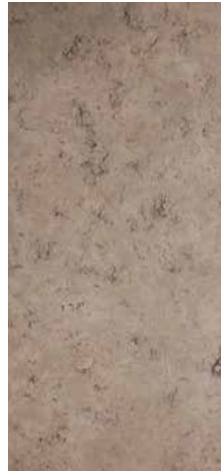
Figure 148. Pavement, DTU Entrepreneurship
