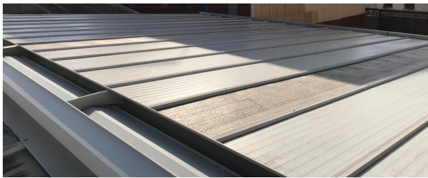
Figure 42. (left) Photograph of an area of the roof of the nave showing the fretwork, skylights and sandwich panels. Source: Own: Own. (right) Section of a typical sandwich panel for roofs. Source: Google Images: Google Images
