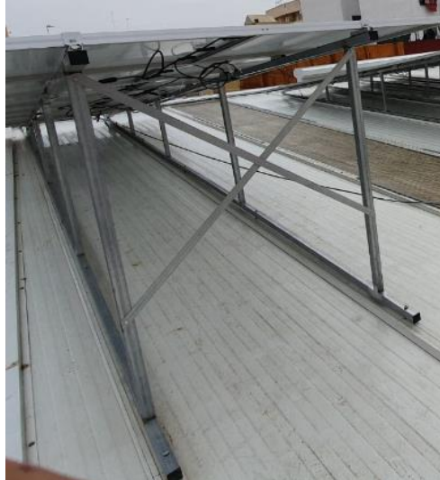
Figure 102. Example of the cross brace for the structure. Source: Own.
