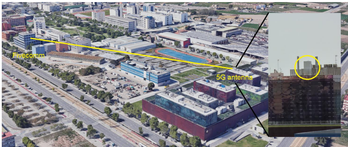
Figure 27 Pointing direction of the mmW antenna installed in the UPV campus
