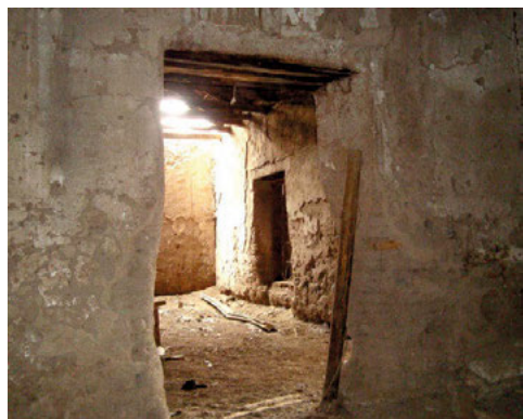
Fig. 1. Casona Quilapilún adobe wall. (Source: Contreras & Jofré, 2016)
