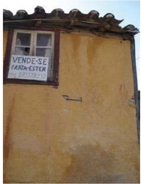
b) Finishing of a tabique wall
