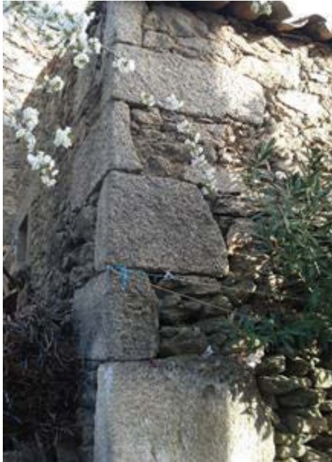
a) Junction of orthogonal walls
