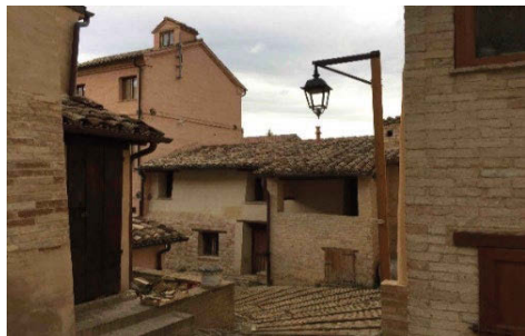
Fig. 3. The village of Villa Finacana in Macerata, after the restoration interventions, 2022.
