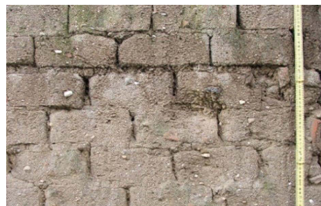
Fig. 4. Earthen wall of a house in the town of Donigala Fenughedu (Oristano) (Source: Putzu, 2015).
