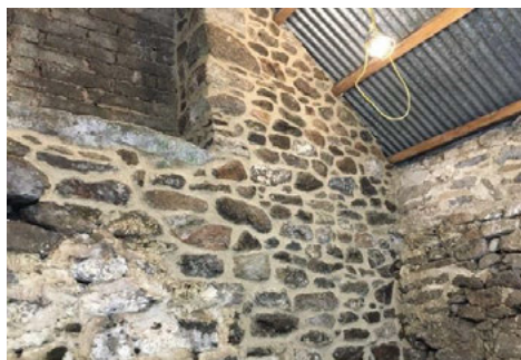
Fig. 8. North side of west gable following rebuilding (Source: Jonathan Rhind Architects, 2021).
