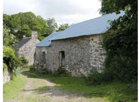
Fig. 5. Pizwell barns (north side) following repairs (Source: White, 2021).
