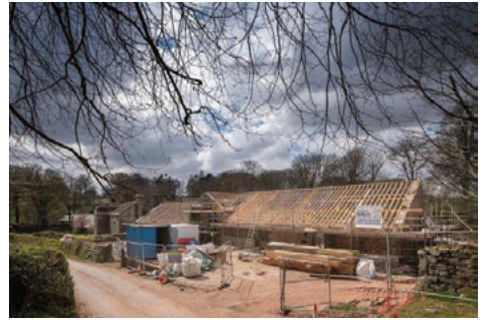
Fig. 11. Great Cator Barn during work (Source: Copyright Historic England Archive, Davies, 2021).
