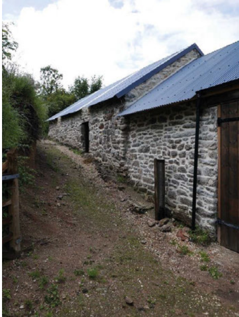
Fig. 10. South wall following repair (Source: White, 2021).
