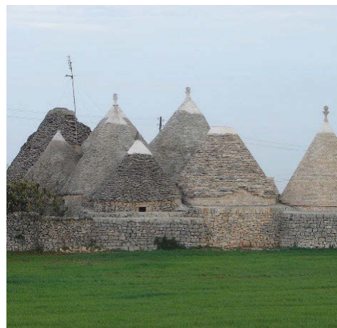
Fig. 3. comparison between original roofs, dismantled and reconstructed roofs and new roofs (Source: Autores, 2008)
