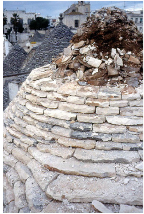
Fig. 8. Bisassembly and reconstruction. (Source: Authors, 2014)
