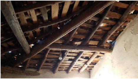
Fig. 7. Roof in Garganta la Olla (Source: Franco, 2020)
