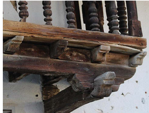
Fig. 5. Balcony in Valverde de La Vera (Source: Franco, 2020)
