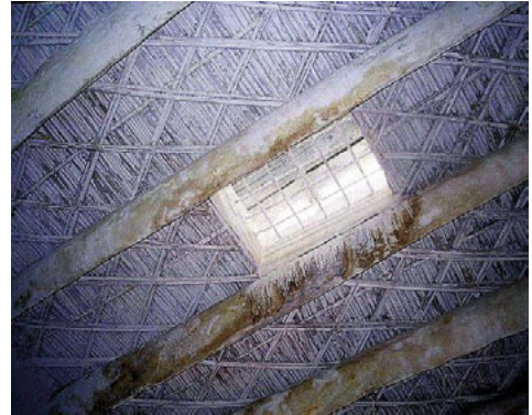
Fig. 4. Traditional Ceiling, ith palm trunks, palm stems and a shaft.
