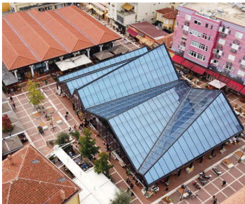
Fig. 2. Tirana Bazaar: photographic image of the current state (Source: Mirra, 2021)
