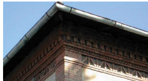
Fig. 2. District San Saba in Rome – brick detail of cornice of one of first 44 houses built between October 1908 and April 1909.
