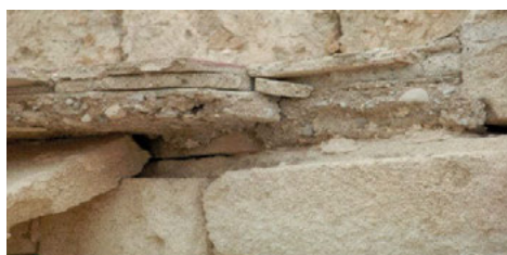
Fig. 19. Layers of the 'realina' tiled vault extrados (Source: Mami, 2018)
