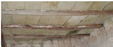
Fig. 11. Timber floor with timpagnoli (Source: Mami, 2018)
