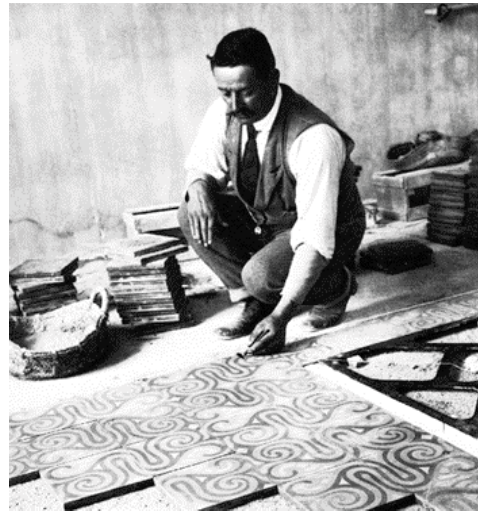
Fig. 10. Installation of Catalanian-inspired hydraulic cement mosaics or tiles. (Source: del Cueto, 2016).
