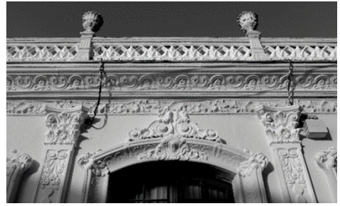
Fig. 9. Ornate façade in Remedios, Cuba using molded cast-stone decoration. (Photo by author 2018).
