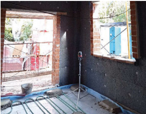
Fig. 8. Insulating by recycled cotton and radiant heat, kitchen area (Source: Li Puma, 2021)
