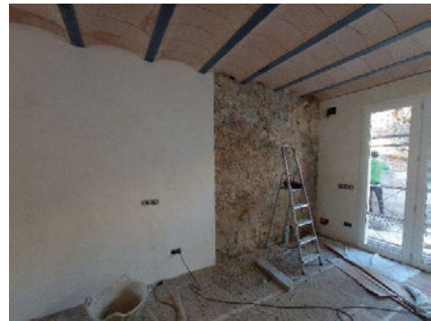
Fig. 6. Cover of interior stone walls, made by calcic lime mortar, leaving parts of uncovered walls (Source: Li Puma, 2021)
