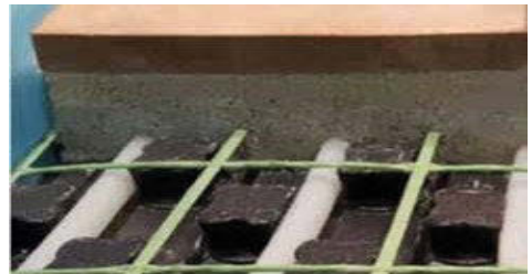
Fig. 9. Radiant heat and clay tiles, detail (Source: “Maestri del Cotto” catalogue, 2021)
