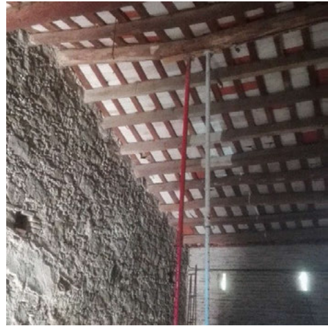
Fig. 2. Original state of the property: interior of the main house in U3, with the wood gabled roof (Source: Li Puma, 2021)
