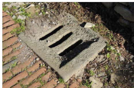
Fig.5. Sandstone storm drain (Source: Fabio Fratini).
