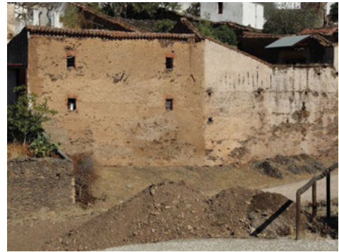
Fig. 2. Housing built with raw earth. Hinojales, Huelva.(Aniceto Delgado Méndez, 2019)
