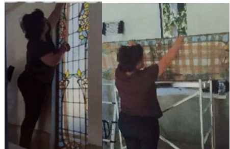
Fig. 8. Disassembly works. British Cemetery (Source: Benavent, 2017).
