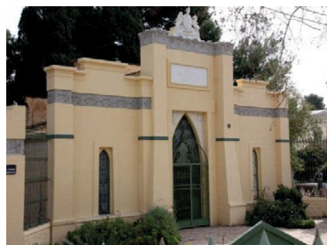
Fig. 1. Façade. British Cemetery, Valencia (Source: Burguete, 2017).
