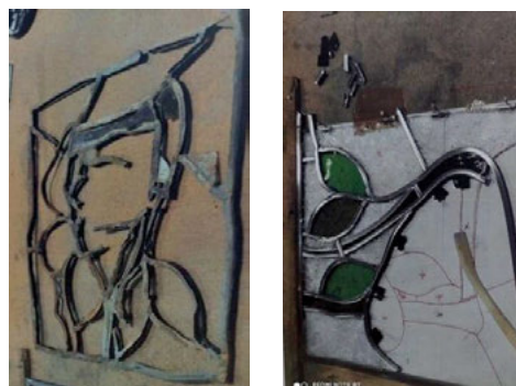
Fig. 11 & 12. Disassembled stained glass lead cord.; stained glass reassembly (Source: Benavent, 2017).
