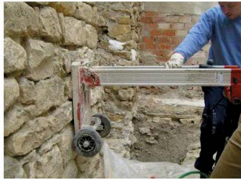
Fig. 6. Test about the internal composition of the façade of the Royal Butchers (16th century) in Porcuna, during the restoration process. It is possible to observe that the façade is characterized by an orderly configuration, instead the “soul” of the wall is composed of filling material without any consistency. (Source: Millán, 2014).
