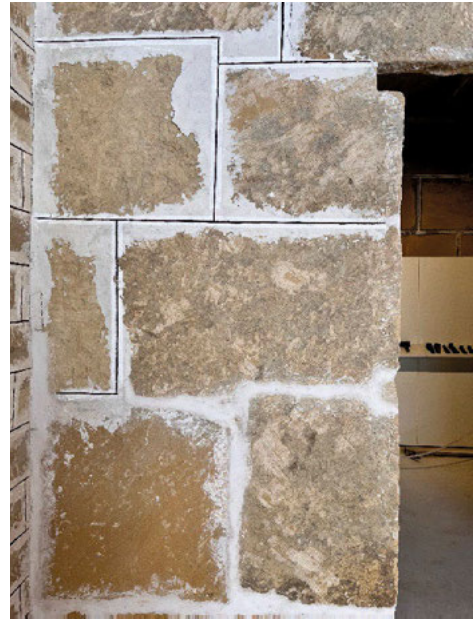
Fig. 5. Detail of a partition wall of losetas (blocks on “sailor” courses). (Source: Belmondo, Millán, 2022).
