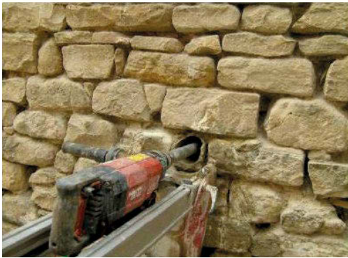
Fig. 6. Test about the internal composition of the façade of the Royal Butchers (16th century) in Porcuna, during the restoration process. It is possible to observe that the façade is characterized by an orderly configuration, instead the “soul” of the wall is composed of filling material without any consistency. (Source: Millán, 2014).
