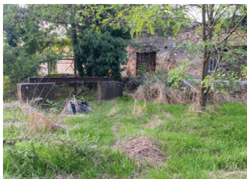
Fig. 8. Benevento, Acqualonga mill. View of the buried canal and of the 20 th century sluice gate.
