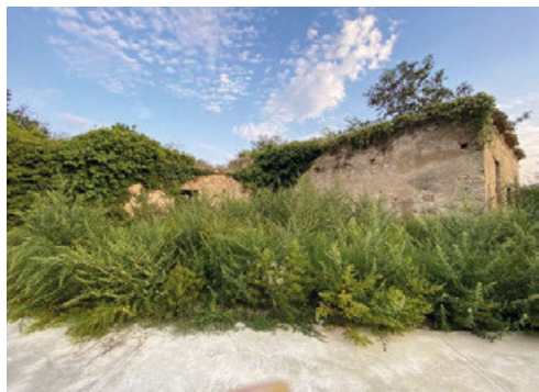
Fig. 7. Benevento, Acqualonga mill. View of the western façade.
