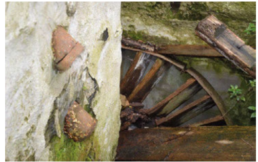
Fig. 12. Benevento, Acqualonga mill. View of the vertical wheel (Source: Cuntò, Intermoia, Longo, 2016).
