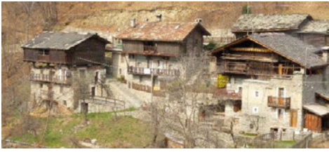
Fig. 4 The main façade in Ayas and in Saint-Vincent.
