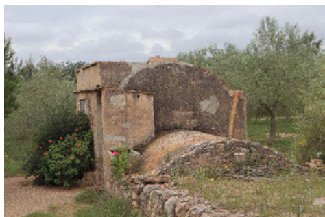
Fig. 6. A cistern covered by ceramic vault (Source: Anna Martínez, 2021)
