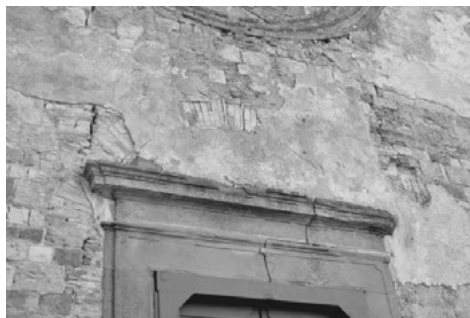
Fig. 6. Exhaust arch. Church of S. Gavino Adimari (Source: Bordini, 2021)
