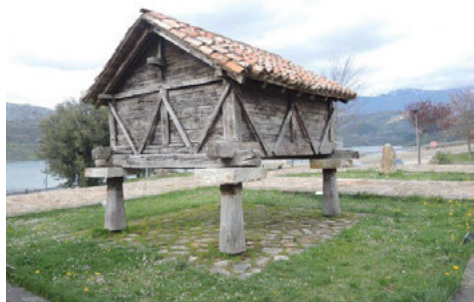
Fig.4. Leonese hórreo from Salio dismantled and remounted in Nuevo Riaño (Source: Pablo Herrero Lombardía).
