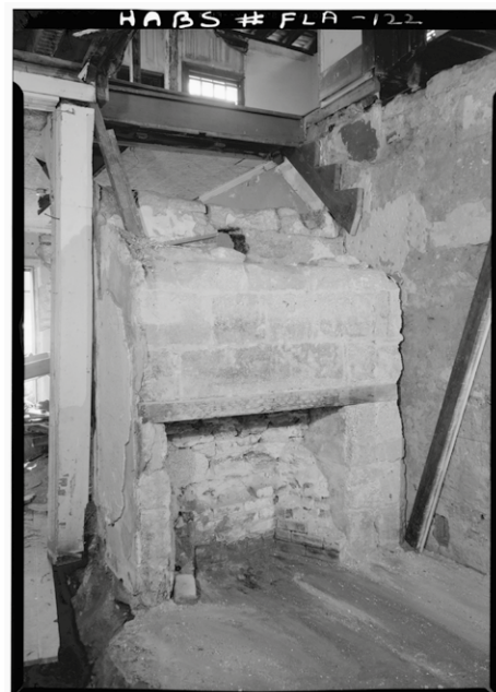
Figura 54: Chimenea planta baja en la restauración de 1960. Fuente: Historic American Buildings Survey, C. (1933) Don Raimundo Arrivas House, 44 South George Street, Saint Augustine, St. Johns County, FL. St. Johns County Florida Saint Augustine, 1933. Documentation Compiled After. [Photograph] Retrieved from the Library of Congress, https://www.loc.gov/item/fl0198/ .
