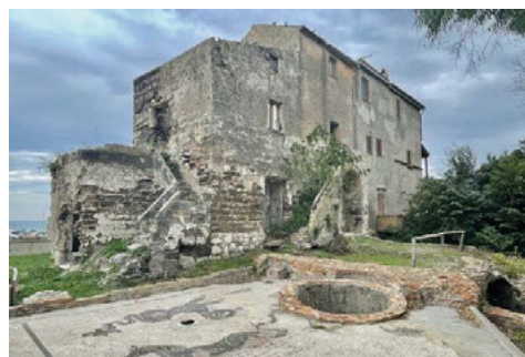
Fig. 1. The rests of the Villa San Limato with the surviving structures of a farmhouse (Source: Cappelli, 2021)
