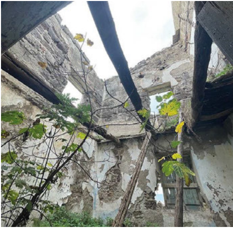
Fig. 8. The wooden beams of the ancient floor of the farmhouse (Cappelli, 2021)
