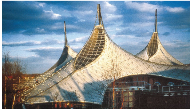
Figure 22. High point with a cable loop in a cable net. German Pavilion. Montreal Expo 1967. ©Atelier Frei Otto + Partner
