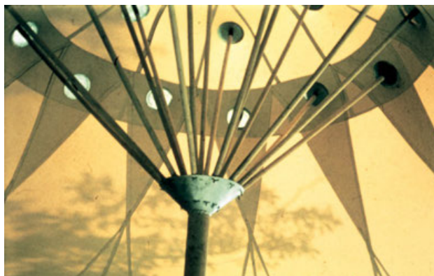
Figure 20. Mast tip split in a bundle of rods. Federal Garden Show. Cologne, 1957. ©Atelier Frei Otto + Partner
