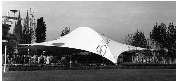
Figure 18. Arch-supported entrance canopy. Federal Garden Show. Cologne, 1957. ©Atelier Frei Otto + Partner
