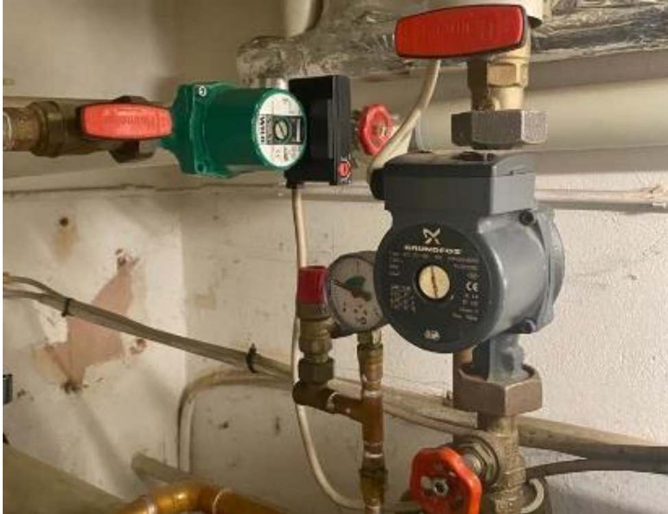
Figure 2.5: Picture of two wet-rotor pumps installed in a heating system
