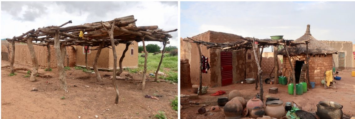
Figure 12. Shed next to the access to a courtyard and inside the courtyard (Cases 1.0. and 4.0.).
