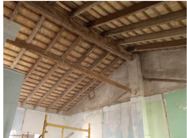
Figure 3 | Traditional roof in Valencian Community
