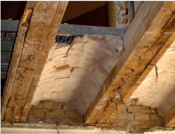
Figure 2 | Jack arch floor in Valencian Community.
