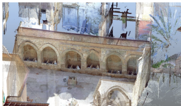
Fig. 10. As-built point cloud of the arcosolium compositional succession of San Juan del Hospital de Valencia. Source: García-Valdecabres et al. (2016).
