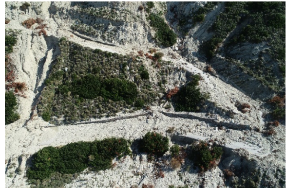
Figure 2. The infrastructure suffered extensive destructions caused by material relocation which resulted severe damage due to erosional phenomena and mudflows.
