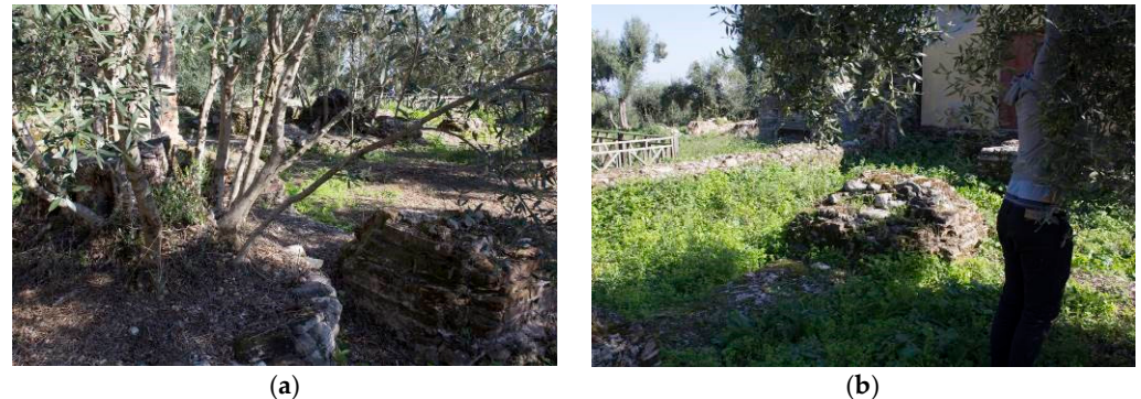
Figure 3. Presence of trees in the site that covered the wall structures (a) and trick used to have a better view of the structures in the images (b) (photo by the authors).
