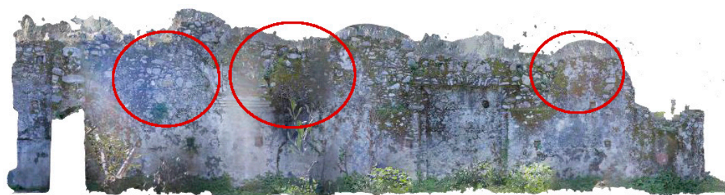
Figure 5. The orthophoto of the southern wall with the prints of the arches highlighted with red circles (authors’ elaboration).
