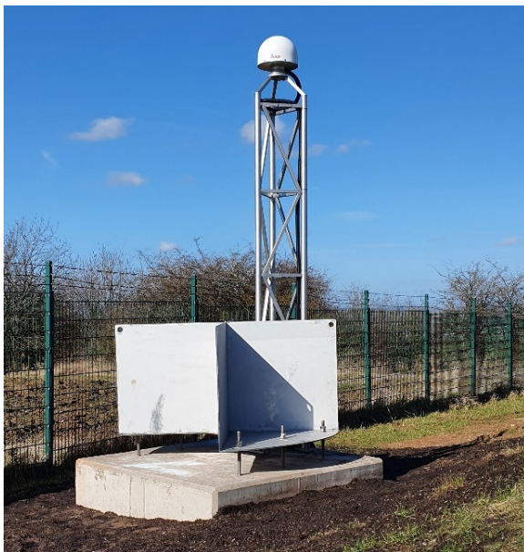
Figure 9. LVGL's MSST Felsberg for Saarland's SAARBOBEKA on a reinforced concrete foundation 2 m x 2 m x 2 m, Leica AR25 GNSS chokering antenna, D-CR Ø2,0m and levelling points in foundation and D-CR. Image courtesy LVGL.
