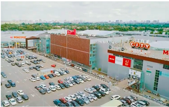
Figure 1. General view of the warehouse.
