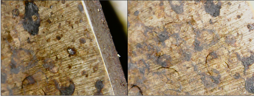
Figure 5.12: Detail of fouling observed on the bypass flap
