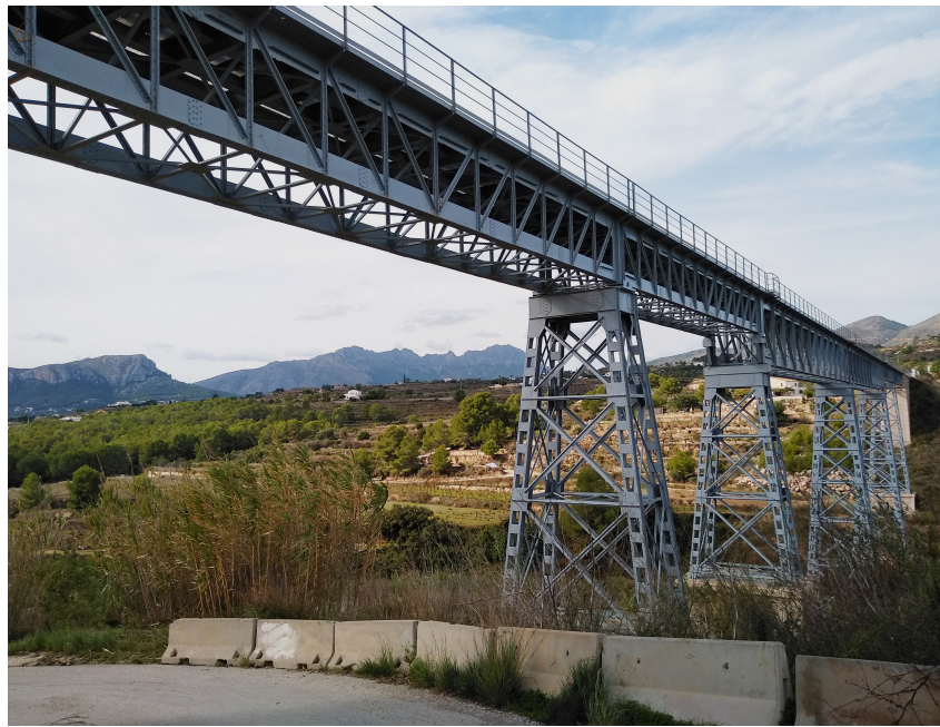
Figure 4.3 Quisi bridge, Benissa, Valencia Region
