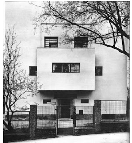
FIG 5. Fachada principal casa Müller
