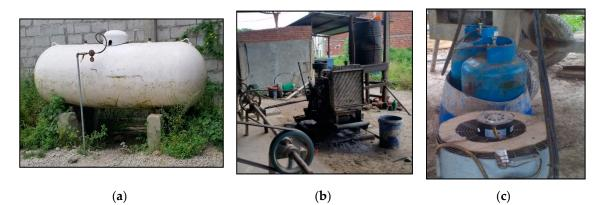
**Figure 9.** Types of fuels used as a heat source: (**a**) liquefied petroleum gas (LPG) tank for industrial use; (**b**) Diesel used for the operation of the generator; (**c**) LPG cylinder for domestic use.
