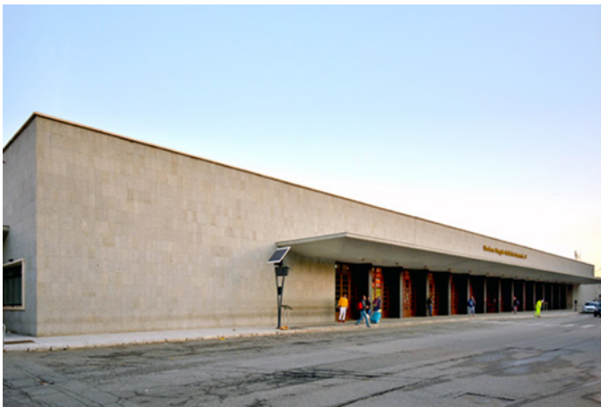
Reggio Calabria. Central Station, Angiolo Mazzoni 1936-1938. On the right, the rehabilitation worksite of the main façade carried out in 2018 and the façade with the new slabs in place. The original marble cladding has been “pulled down, demolished and thrown away” (left and right down photos by R. Castiglia, right up [8]).
