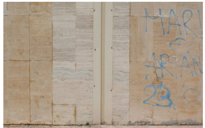
Messina. Central and Maritime Station, Angiolo Mazzoni 1934-1940. On the right, a detail of the original Alcamo travertine slab cladding compared with others replaced during the maintenance work carried out (1960-2000 span). (Photos by A. Cernaro).
