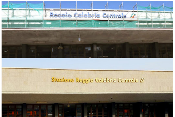
Reggio Calabria. Central Station, Angiolo Mazzoni 1936-1938. On the right, the rehabilitation worksite of the main façade carried out in 2018 and the façade with the new slabs in place. The original marble cladding has been “pulled down, demolished and thrown away” (left and right down photos by R. Castiglia, right up [8]).
