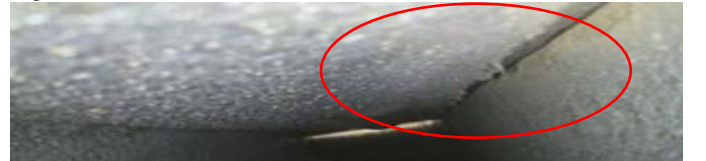
Fig. 4. Mechanical Erosion (2014) – Slot No 14 – Ventilation Channel No 01 Top Side Out.
