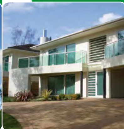
PLC (power line communication)
